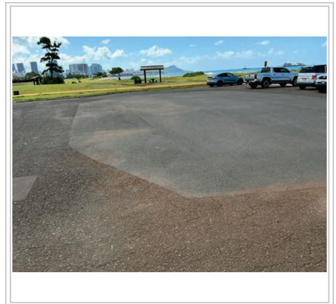
Area to be repaved
