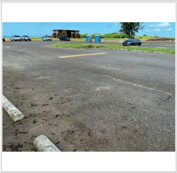
Area to be repaved
