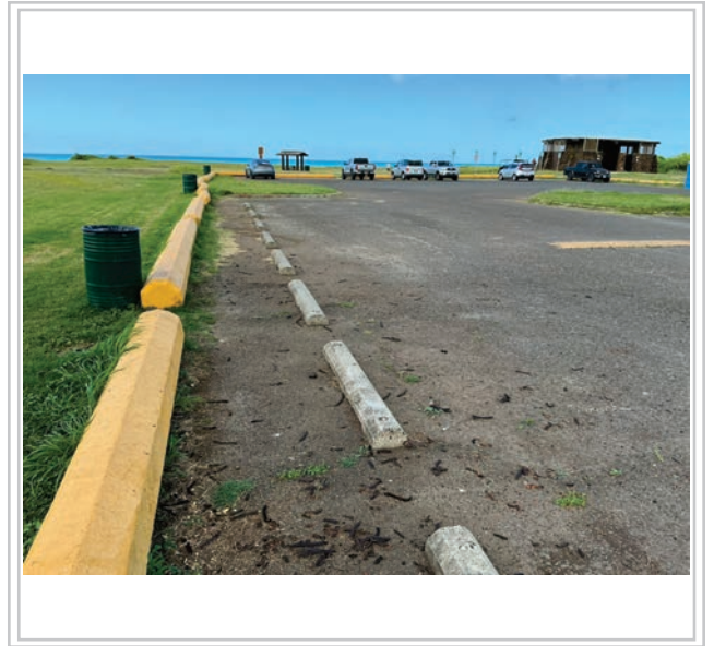
Area to be repaved
