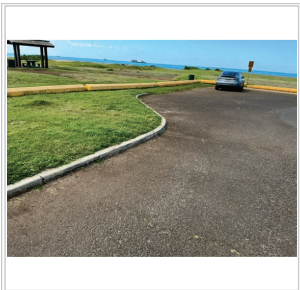
Area to be repaved
