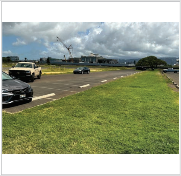
Area to be repaved
