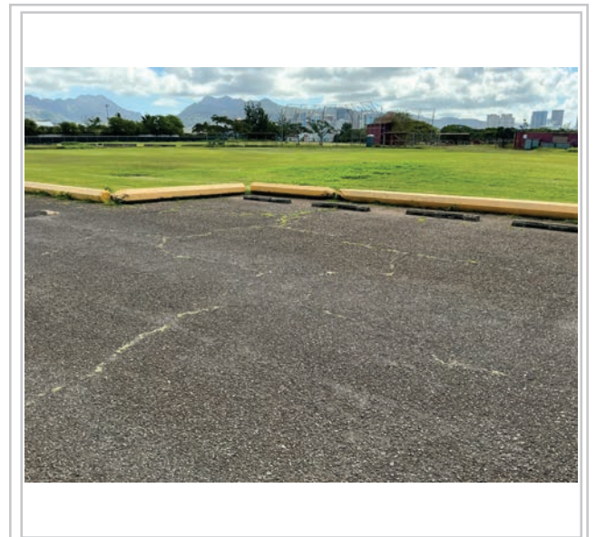
Area to be repaved
