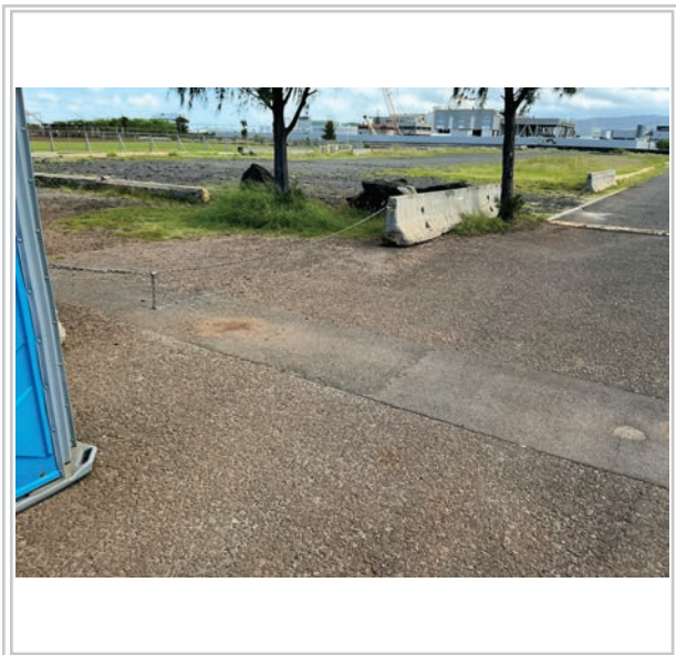
Area to be repaved
