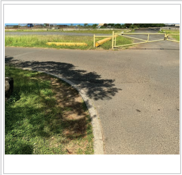
Area to be repaved
